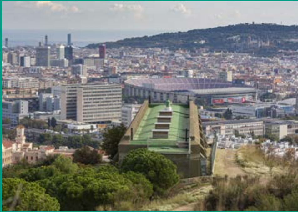
Finestrelles water tank. © Quim Roser
