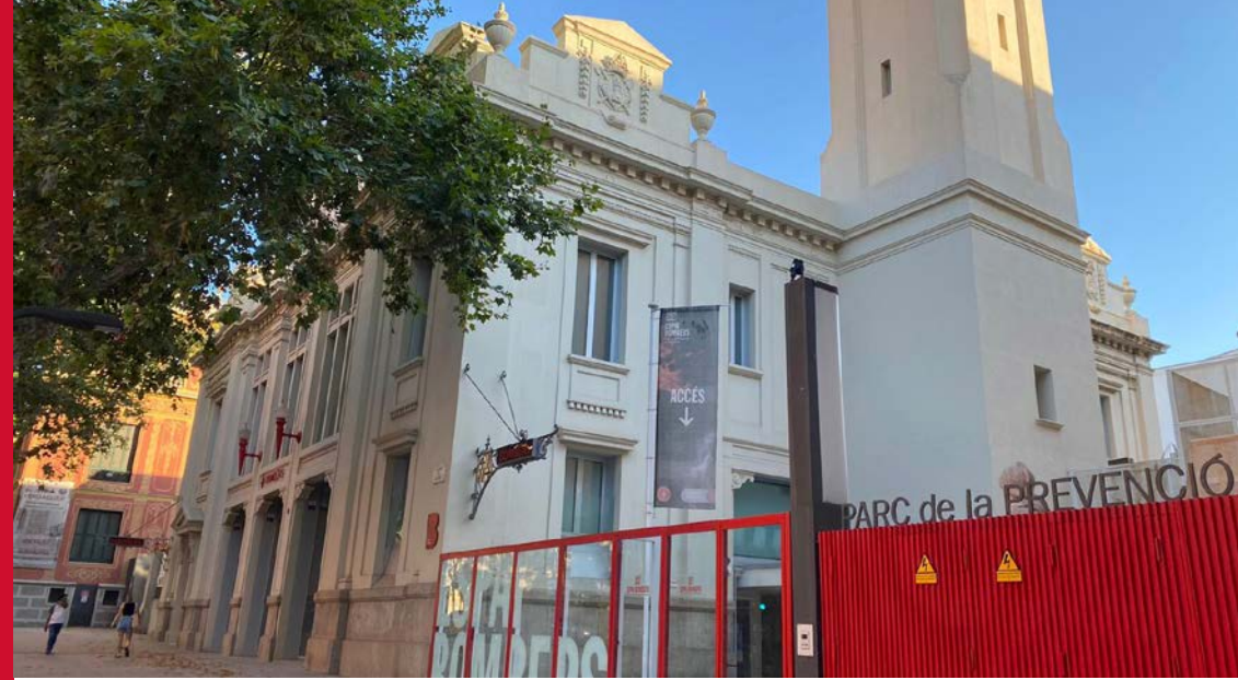
Espai Bombers. Prevention Station on Lleida Street opened in 2016.
