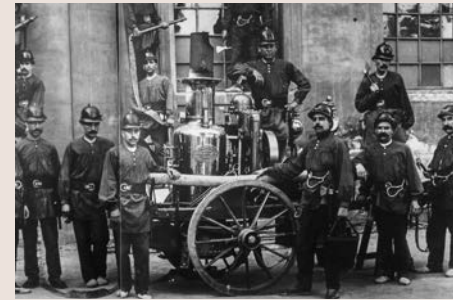
Merryweather Valiant II 1896. Bought in 1896. Made in the UK. Light steam pump with a 900 l/m flow rate. At least two firefighters were needed to move it around. ABB
